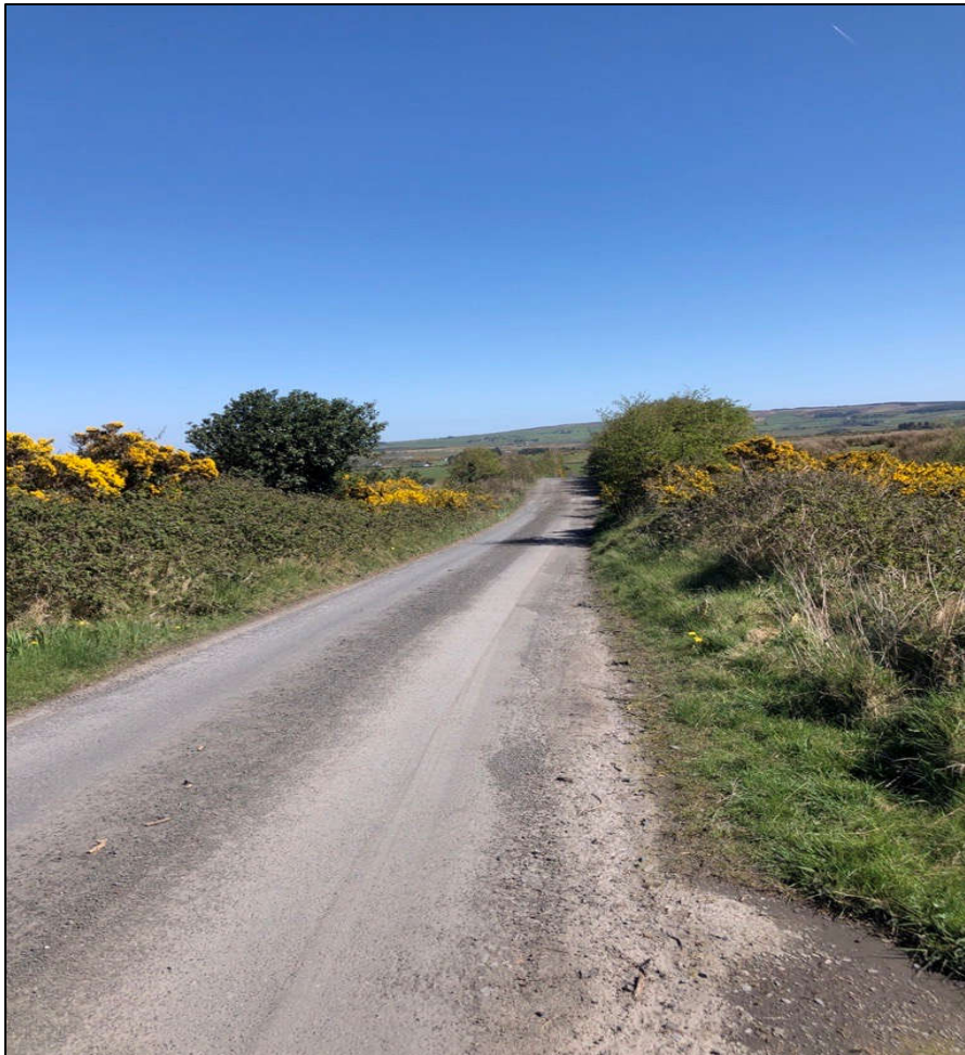
Plate 6-16 Existing Road (BL3) into which the cable is going to be laid.
