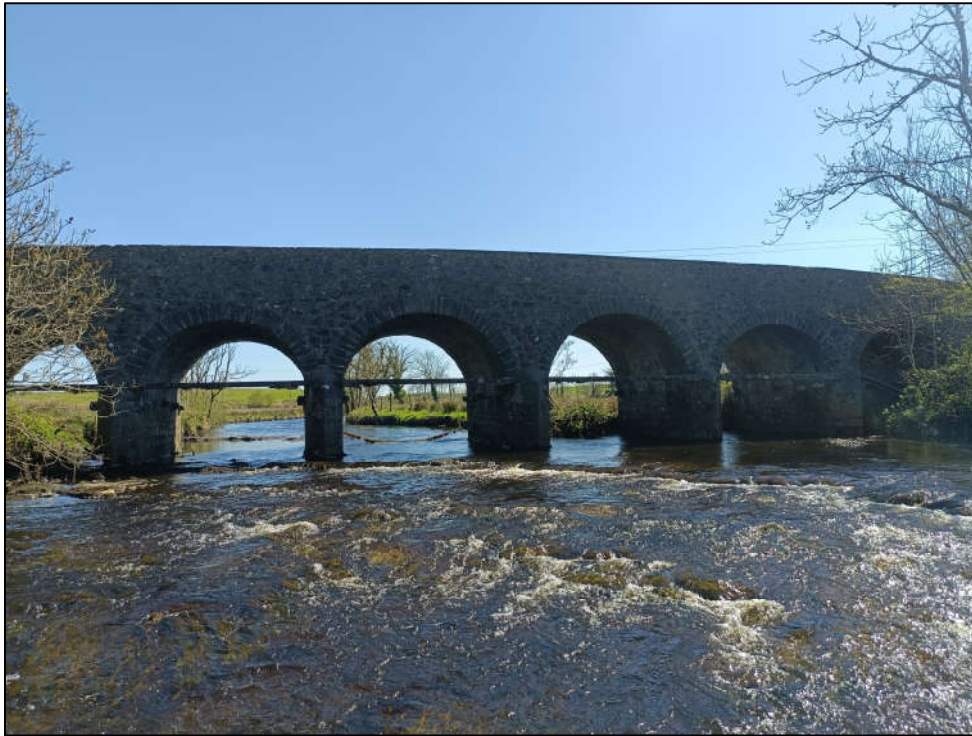
Plate 6-17. Cloonaghmore River along the Grid connection route
